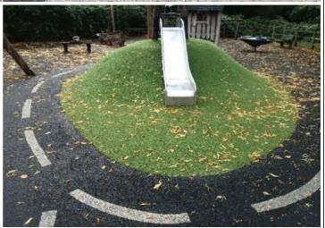
Finding: There is some damage to the wet pour surfacing
