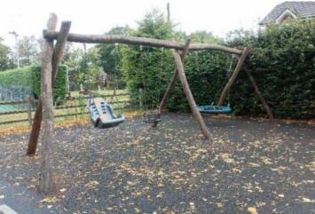
**Finding:** This design of swing joint has been known to fail on the weld connecting the joint to the threaded stud
