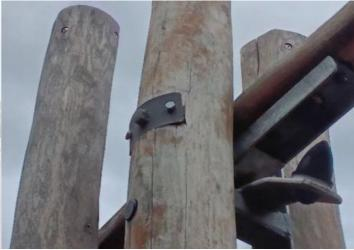
Finding: The fixings are not flush with the fixing plate
