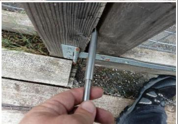
**Finding:** There are gate openings that are less than 12mm that could trap or crush fingers **Action:** Provide a 12mm gap throughout full range of motion at both sides of gate
