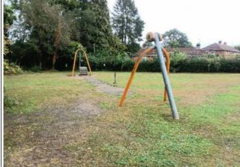
**Finding:** The cable stop above the start ramp is likely to encourage users to lean off the back of the platform
