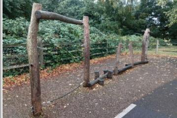
**Finding:** There is or are fixings missing on the rotating beam
