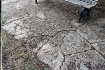
Finding: There is moderate damage to the concrete pad
