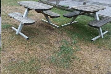
**Finding:** The table/s is/are not secured to the ground and there is some potential for the item/s to be moved within falling spaces of equipment
