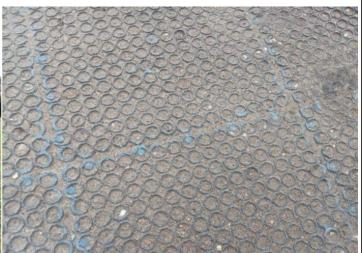
**Finding:** Hard fixing pins have been installed in the grass mat tiles within the impact area of the equipment. Grass mat pins should only be installed at the perimeter of the tiles, and outside of any equipment impact areas. NOTE - where grass mat wear pads have been provided and the impact area includes surrounding surfaces, the grass mats should be tucked into the turf, and not pinned
