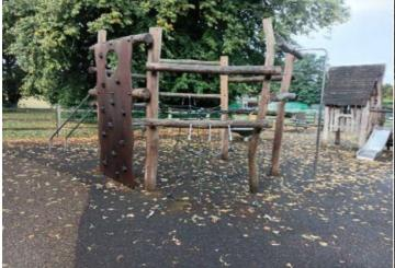
**Finding:** There is/are finger entrapment/s in the climbing panel and the item fails to meet the requirements of BS EN 1176 Part 1 4.2.7.6 Entrapment of fingers
