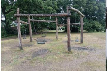
**Finding:** There is algae or moss on the surface of the equipment that can lead to the onset of rot
