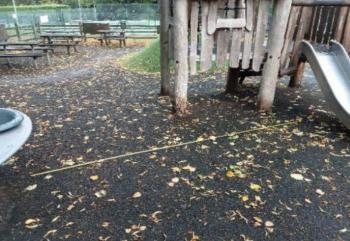
Finding: The free space overlaps the falling space between Action: Monitor - No remedial work recommended the roundabout and adjacent equipment in contravention of the requirements of BS EN 1176:2017 Part 1
