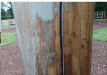
**Action:** Monitor and ensure any rough or splintering edges are sanded down
