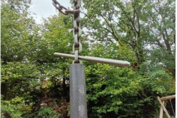
**Finding:** The chain openings are in excess of the 8.6mm as **Action:** Monitor - No action given the risk assessment recommended by BS EN 1176
