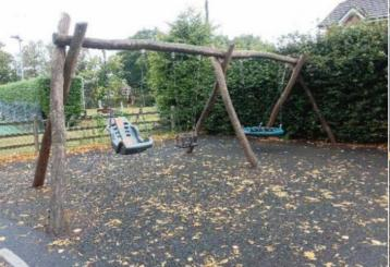
**Finding:** NOTE: The inclusive seat is particularly high at 800mm which may make access and egress difficult for smaller users (We recommend a seat height of 400-500mm)
