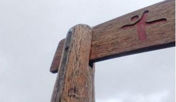
Finding: A number of mast fixing(s) have worked loose
