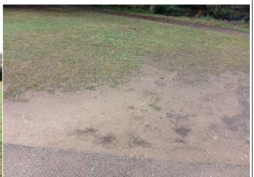
**Finding:** The surface has eroded in some areas and may be **Action:** Reinstate the surface slippery in wet conditions
