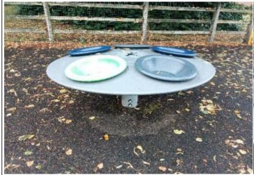
**Finding:** The multi-play forms a projecting obstacle / hard object within the falling space of the equipment, in contravention of the requirements of BS EN 1176 Part 1
