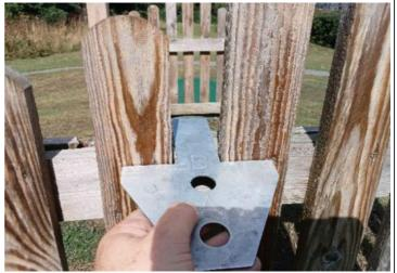
**Finding:** The item fails to meet the requirements of BS EN Action: Monitor - No action given the risk assessment 1176 Part 1 4.2.7.2 for head and neck entrapment in the barriers
