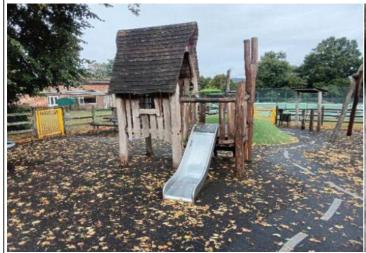
**Finding:** The use of synthetic fillers in timber is not recommended; timber being a natural material will expand and contract as the moisture content changes and the use of fillers can exacerbate the length and depth of these cracks or shakes in the timber. The only treatment that is normally required is the removal of any rough or sharp edges unless the structural integrity of the item is affected.
