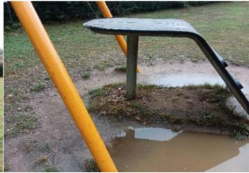
**Finding:** The grass has eroded within the impact area of the **Action:** Reinstate the grass or provide an all weather equipment and may not provide the necessary impact surface attenuating properties for the equipment fall height; the surface may also be slippery in wet weather
