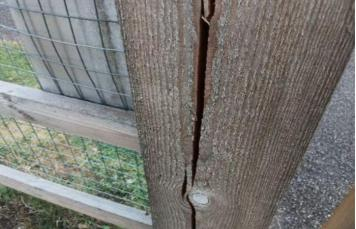
Finding: The timber has a number of splits/shakes or air cracks and this may affect the stability or allow water ingress the splits do not cross through fixing points of the structure which will accelerate the rotting process. Timber splits may and/or cause any instability also create rough / splintering edges.
