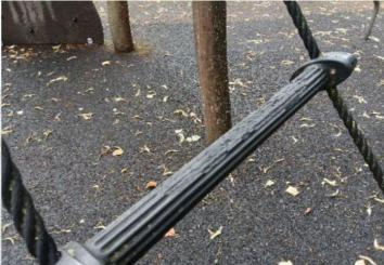
Finding: The rope ladder tread has been damaged
