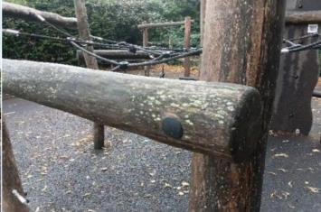
**Finding:** There is algae or moss on the surface of the equipment resulting in slippery conditions
