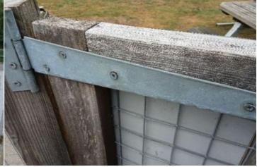
**Finding:** A number of gate hinge fixing(s) have worked loose
