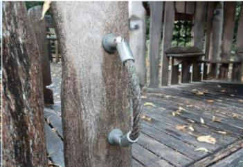
Finding: A number of handgrip fixing(s) have worked loose Action: Secure all loose fixings
