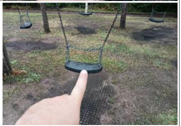
**Finding:** The chain links are worn excessively (50%) and require renewing
