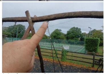
**Finding:** A number of crossbeam fixing(s) have worked loose
