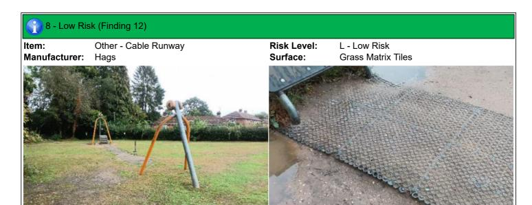
**Finding:** The surface is lifting at the edges and creating trip **Action:** Repair perimeter of surfacing to remove trip points points
